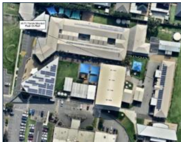
100kw of Solar Panels on the Lighthouse buildings
